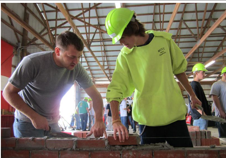
Adam Johnson, Springboro, Senior Heavy Equipment, tries his hand at masonry
